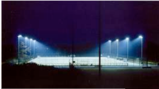
Upton Leisure Centre, Chester (Abacus Lighting)
