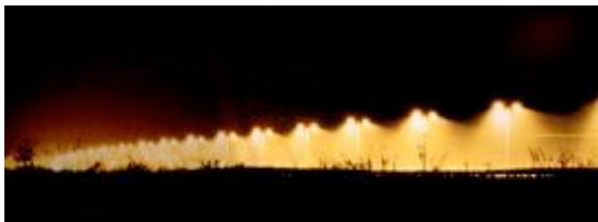
Full cut-off motorway lights
