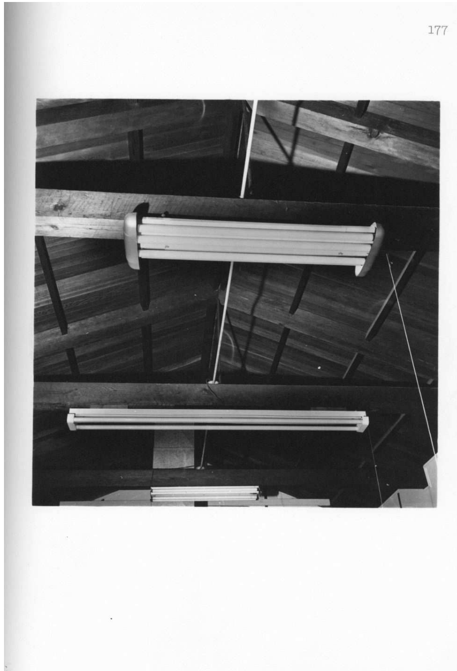
Figure 4.8: She peaked roof of the Central Room of the Playbox. The fluorescent fixtures are attached to three massive cross beams. Brown mounted his baby spotlights on these three beams.
