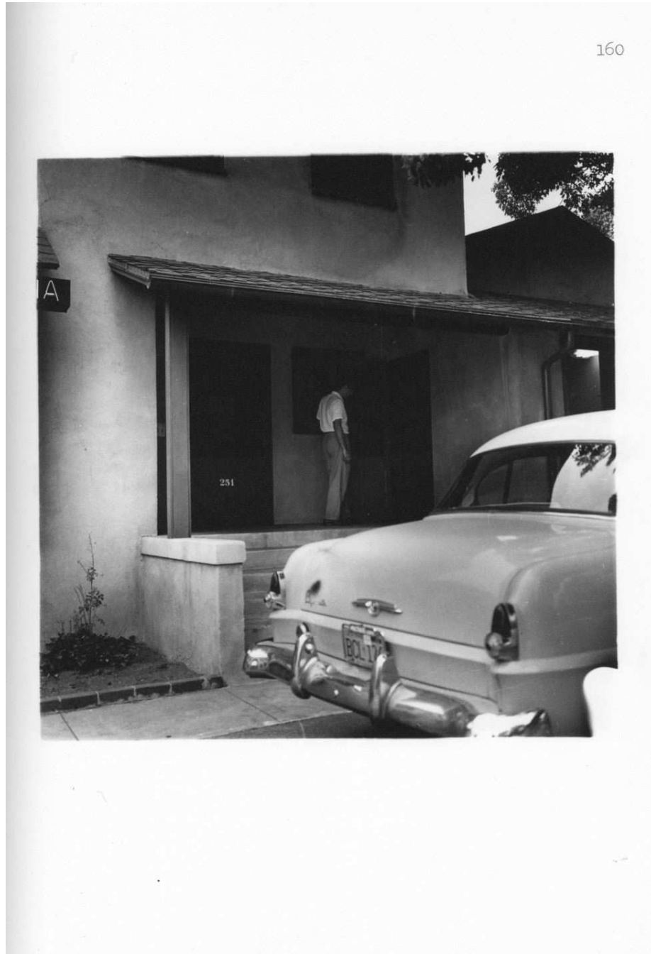
Figure 4.3: The Fair Oaks Playbox building. The front porch. The door at center leads into the entry hall. The door at right leads into the East Alcove.
