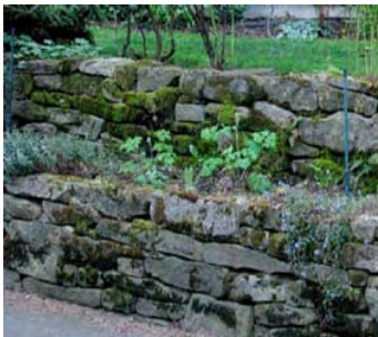
Figure 5.14 - Stepped Retaining Wall
