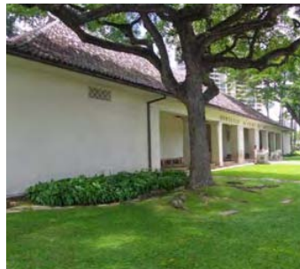
Figure 5.15 - Textured Stucco Wall
