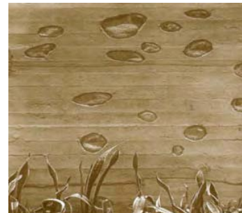
Figure 5.13 - Concept Wall with Exposed Aggregate
