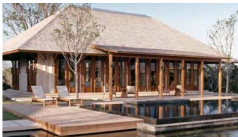
Figure 5.17 - Stained Wood Windows and Doors
