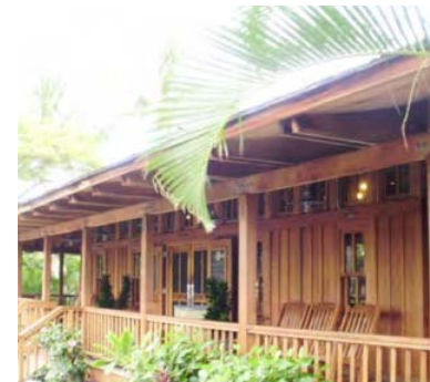
Figure 5.3 - Cedar Board and Batten
