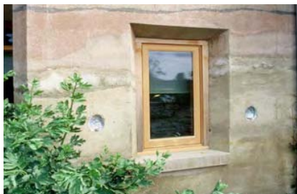
Figure 5.19 - Stained Concrete Wall with Window System Recessed from Exterior Face
