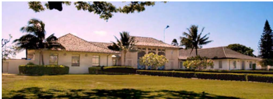
Figure 5.7 - Larger Element in Center of Building Mass
