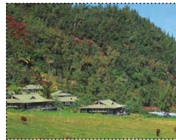
Figure 5.20 - Roof Material and Color Blending in with the Site
