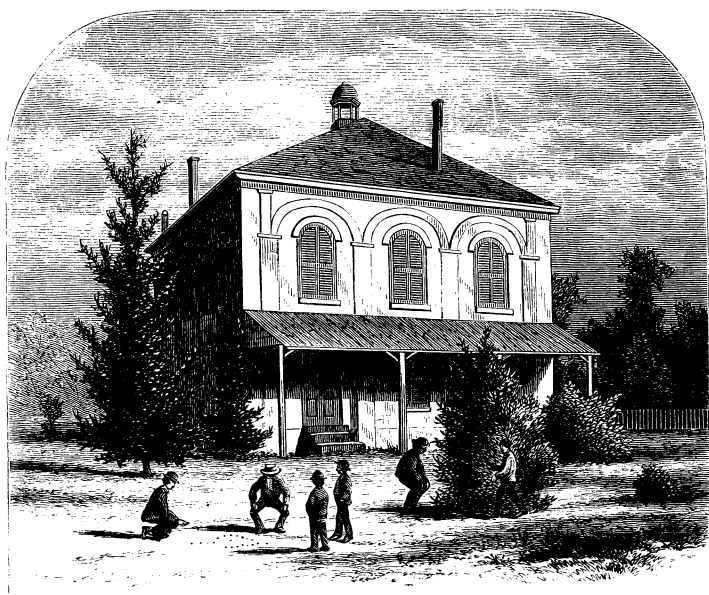
SCHOOL-HOUSE AT ZOAR.
