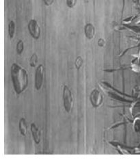
Figure 5.13 - Concept Wall with Exposed Aggregate
