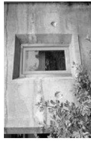
Figure 5.19 - Stained Concrete Wall with Window System Recessed from Exterior Face
